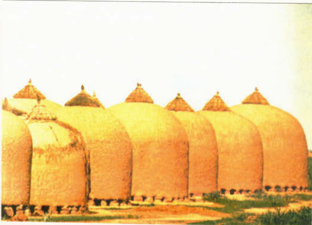
Photo 5: Granaries, with thin mud walls, built with earth and organic fibre.
