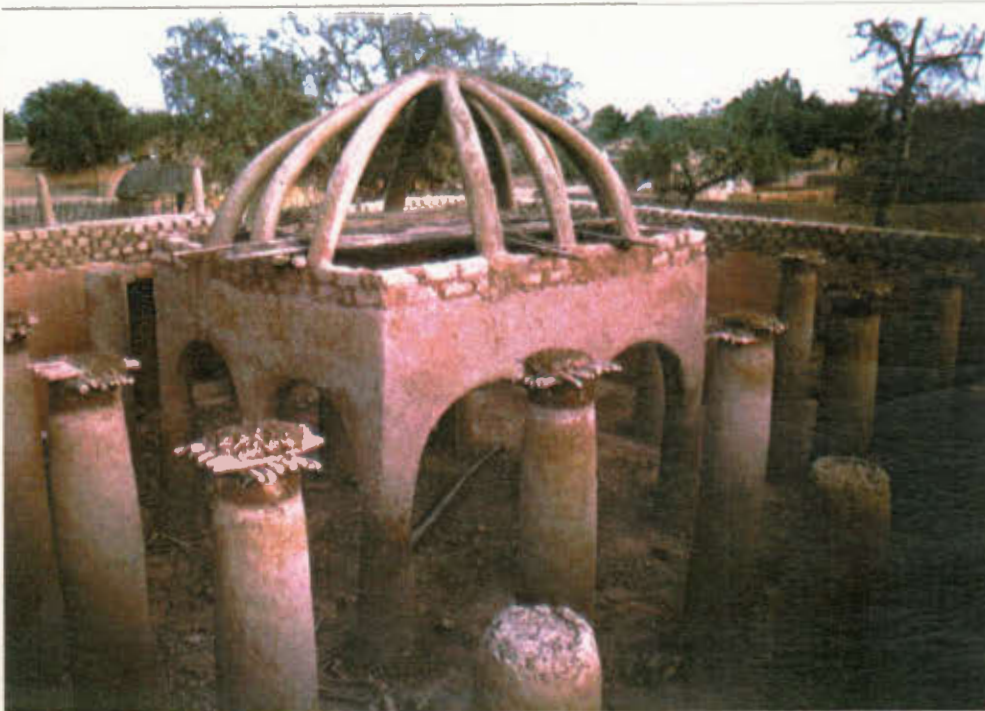
Photo 4: Wooden armature of traditionally built domed building.
