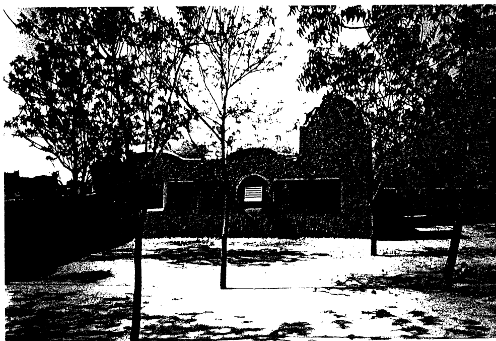
Photo 3: Literacy centre, Chikal, built 1980 in the course of the original training programme introducing the Nubian system for shutterless vault and dome construction in unstabilized sun-dried earth bricks.
