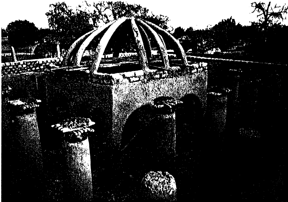
Photo 4: Wooden armature of traditionally built domed building.
