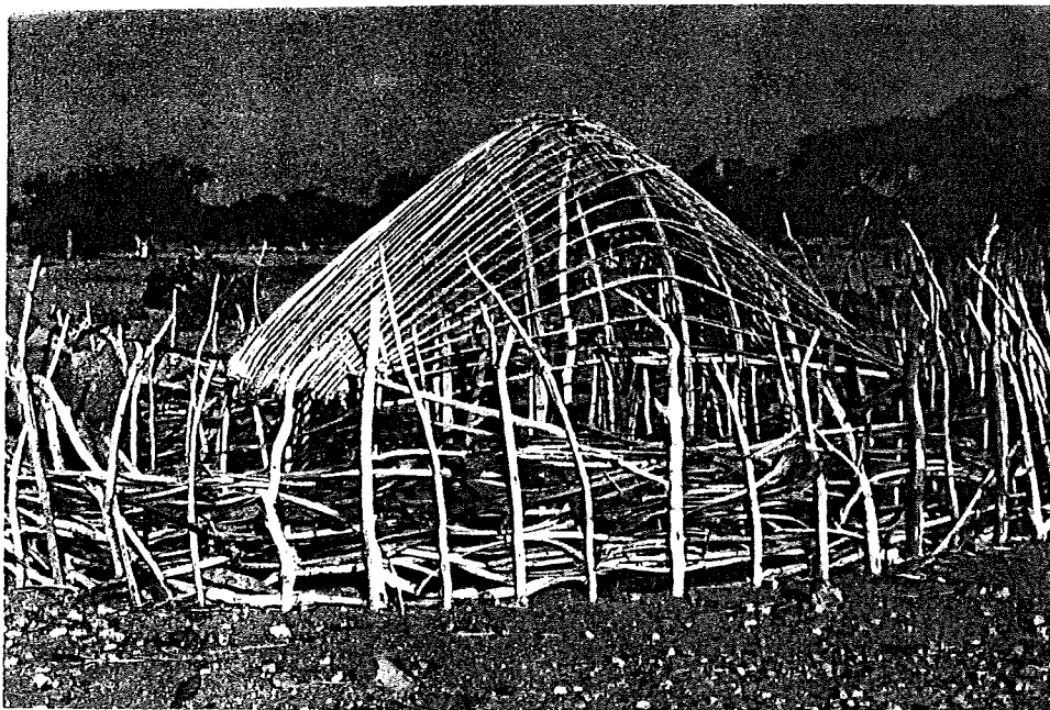
Photo 1: Supporting structure for nomad's traditional tent, Tin Telloust.
