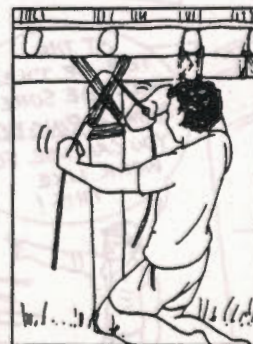
USE WIRE OR BUSH ROPE TO TIE WOOD BEAMS TO FOUNDATION POSTS
