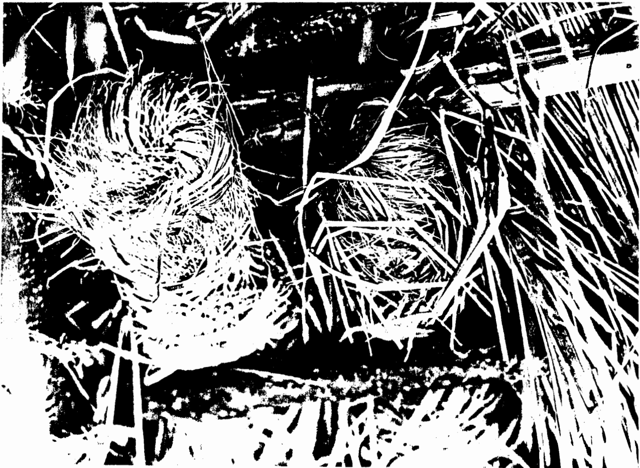
Detail of the bound tops of rice thatch bundles, with supporting battens.
