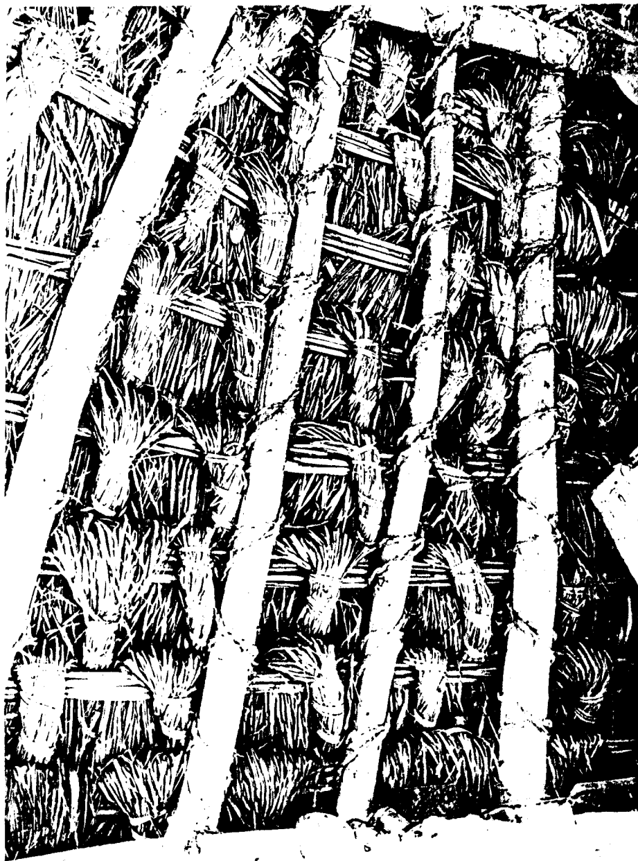
Internal detail of reed thatch showing bundles pulled over battens and tucked behind battens below.
