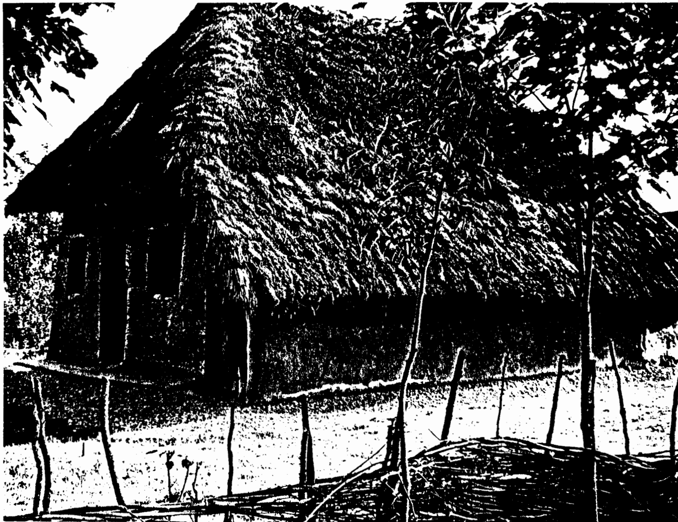
New thatched house with packed mud walls.
