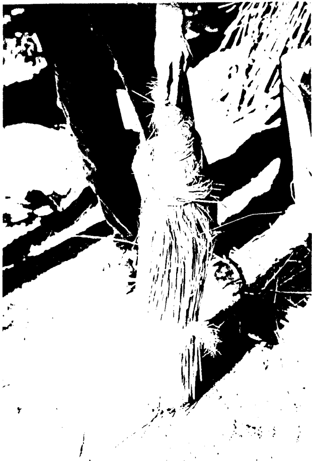
Bundle ready to be passed to roofer.
