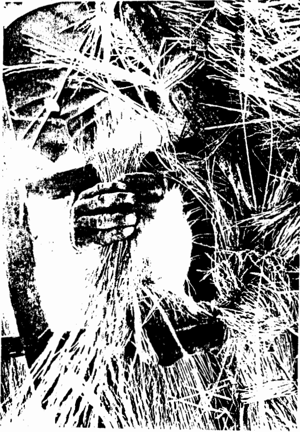
Rice stem thatch in the Shanderman area is tied to battens. These photographs show the process, looking up from the underside of the roof.
