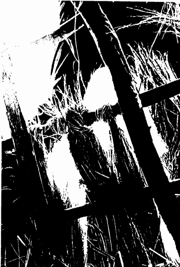
Rice stem thatch in the Shanderman area is tied to battens. These photographs show the process, looking up from the underside of the roof.
