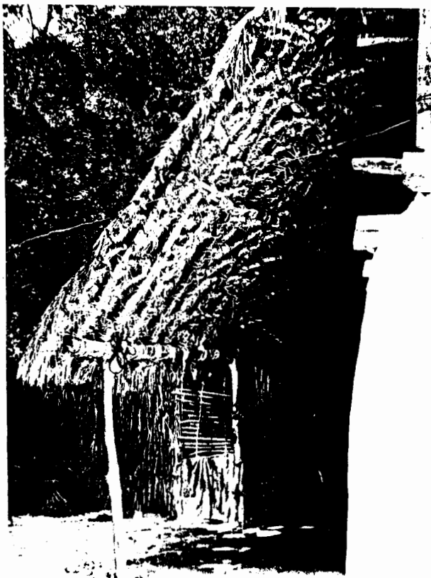
Detail of the bound tops of rice thatch bundles, with supporting battens.
