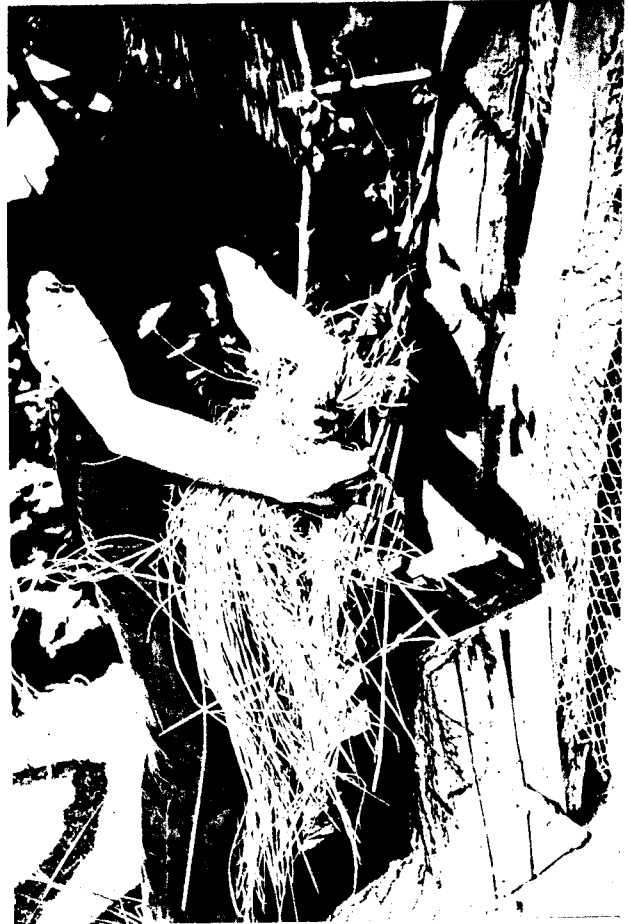
Projecting stems are pulled down and bound round top of bundle.
