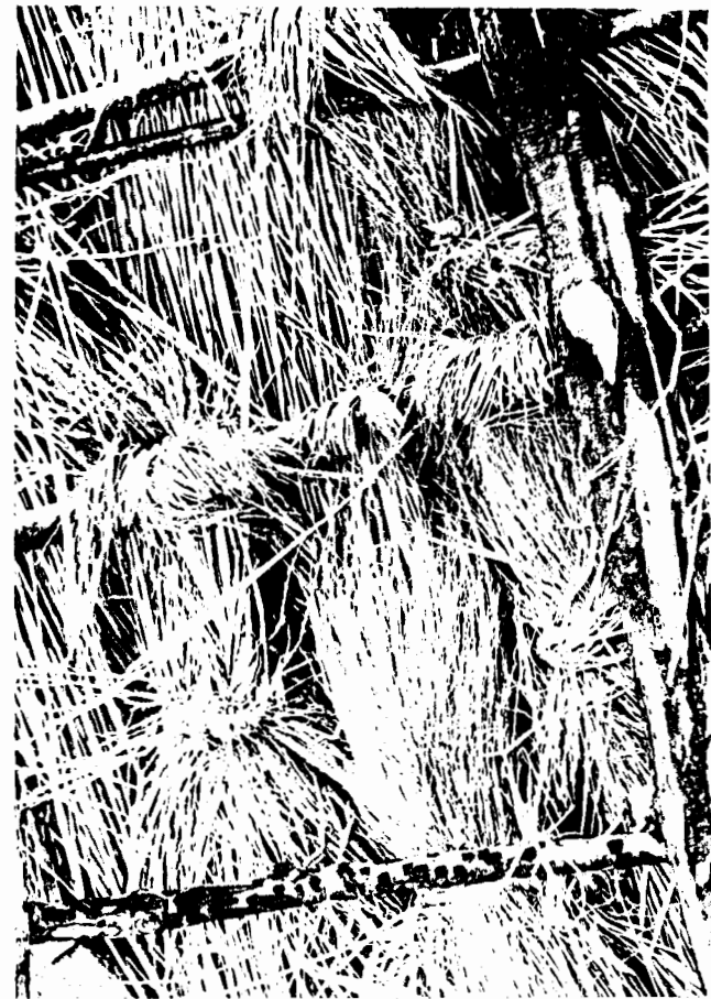
Rice stem thatch in the Shanderman area is tied to battens. These photographs show the process, looking up from the underside of the roof.
