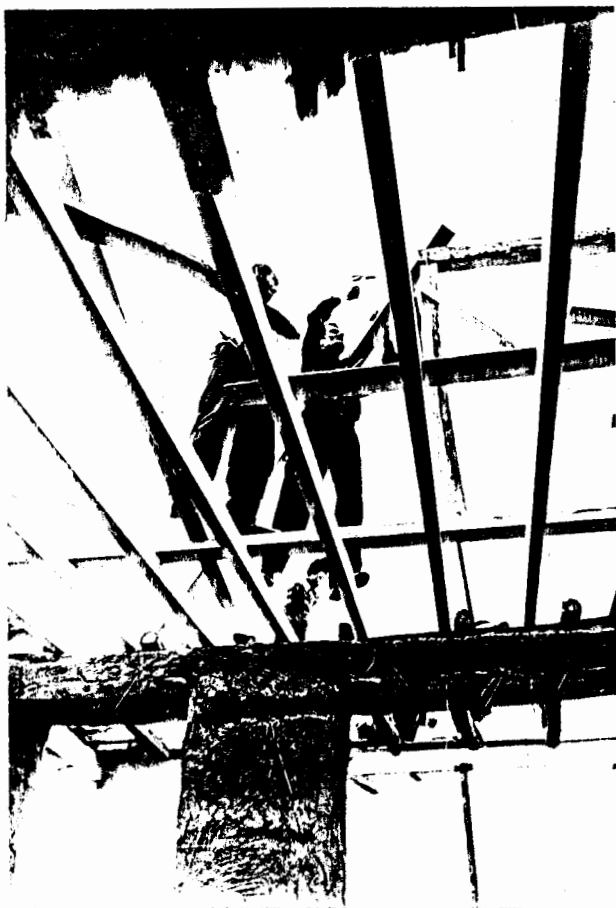
Ceiling joists support the roof framework.
