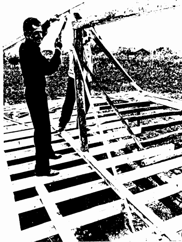
Sheet metal roof trusses are simple. Bracing provides stability during construction and later life.
