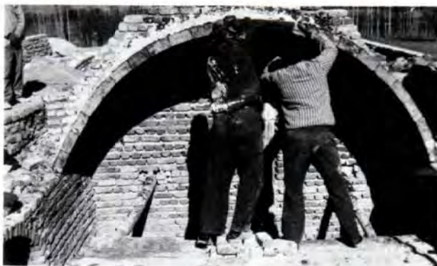
Vault and dome construction can provide inexpensive roofing.
