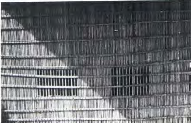
Exterior view of palm frond stem screen. The interior appears to be totally dark giving privacy (Oman)
