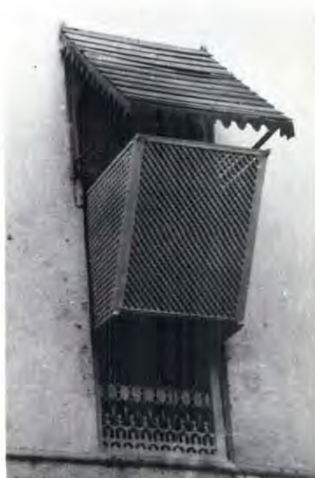
Window mounted evaporative cooler in Muscat, Oman
