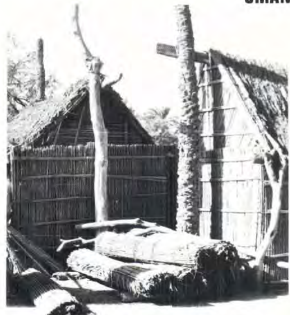
Houses built completely with palm stems. Rolled panels are for use when required.
