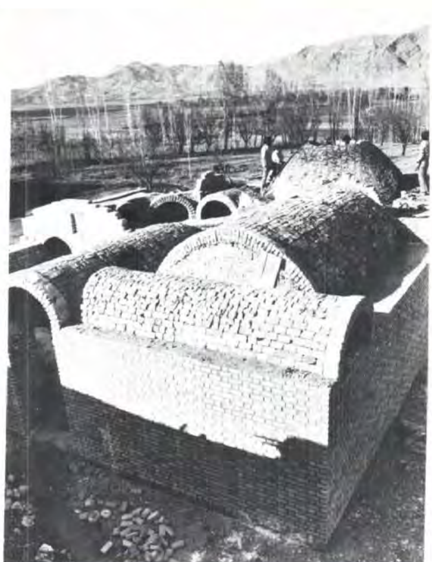
One dome nearing completion. The arches to support the second dome can be seen behind the vaults in the foreground.
