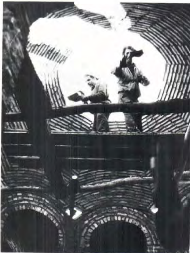
Dome being built over bathroom
