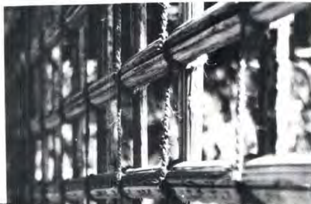
Palm frond stem detail. A smooth transition between light and dark is achieved by the curved section of the material.
