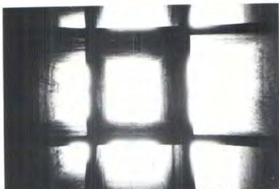
Looking up the tower of a multiple shaft windcatcher in Yazd, Iran. More shafts lead to openings on a particular side to allow increased air movement from a specific direction.
