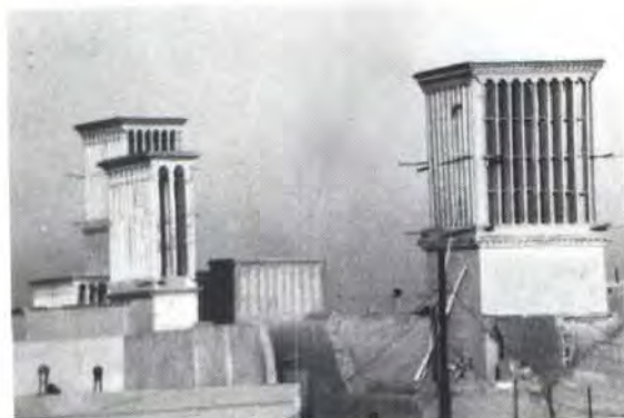
Elaborate windcatchers in Yazd, Iran, with multiple shafts.
