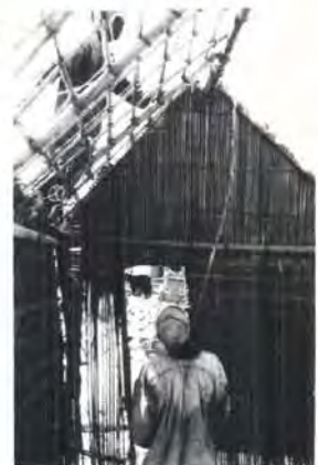
Tensioning framework for palm frond house.
