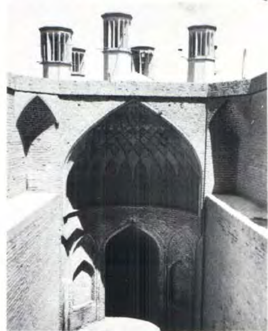
Six windcatchers used to cool an underground water cistern in Yazd, Iran.
