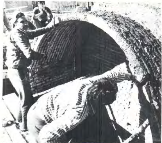
Vault construction over clothes/baby washroom
