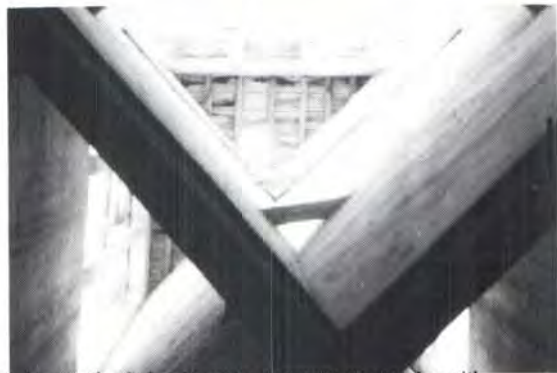
Looking up the shafts of a multi directional windcatcher with 'X' pattern divisions
