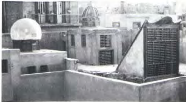
Single directional windcatcher in Cairo, Egypt.
