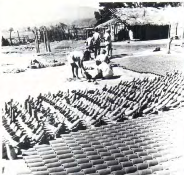
Roof tile making
