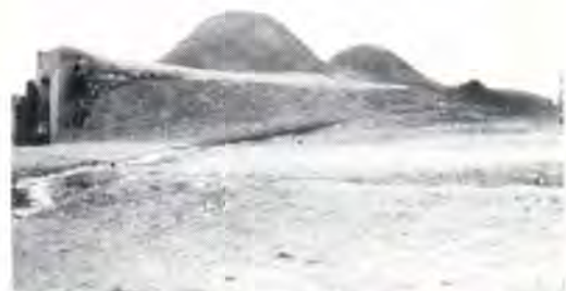
Raised entrance and the domes over the changing and bathing rooms are the only visible part of many traditional baths. Baths are below ground level for insulation and to allow water supply to flow by gravity.
