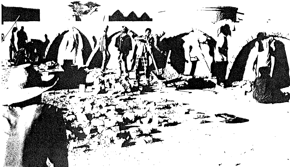
Photo 7: Training programme, Iférouane: practising vault building.
