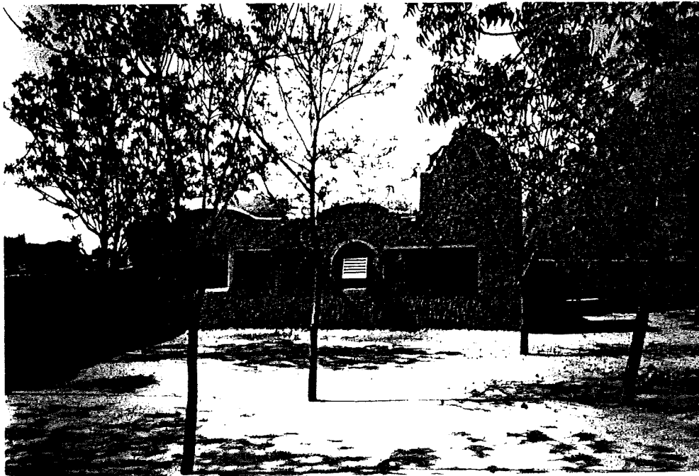
Photo 3: Literacy centre, Chikal, built 1980 in the course of the original training programme introducing the Nubian system for shutterless vault and dome construction in unstabilized sun-dried earth bricks.
