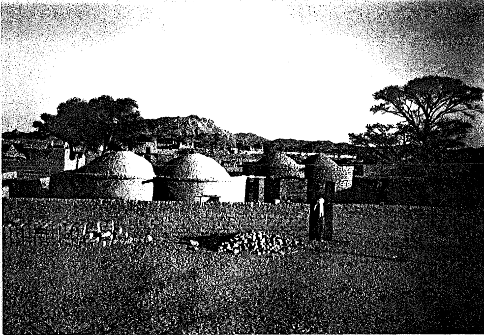
Photo 13: Private houses (2 round rooms, with domed roofs) built by Moussa Amgar and his team, Iférouane. (For actual costs of these buildings, see page 32, House type 2.)
