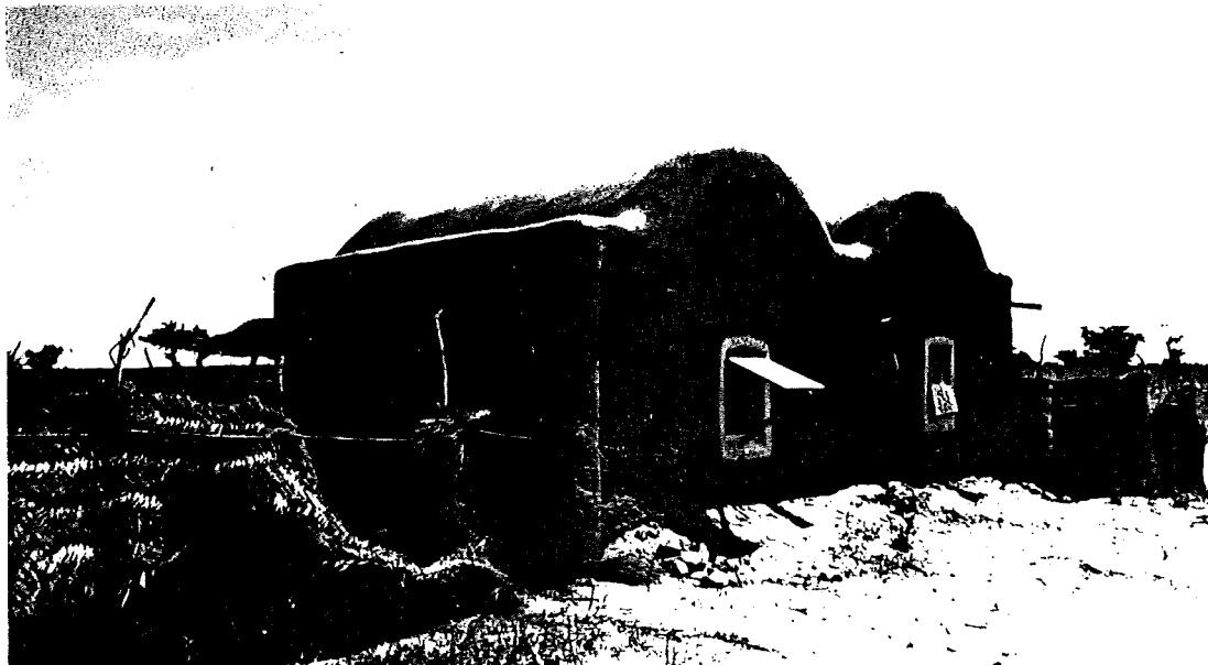
Photo 22: Two-room house with vaults; see page 32, House type 3, for actual costs of this building.
