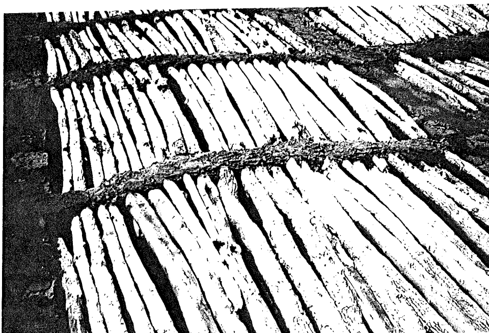
Photo 2: Recently constructed roof consisting of wooden beams and rafters, seen from above, before covering with mats and earth; south of Agadez.
