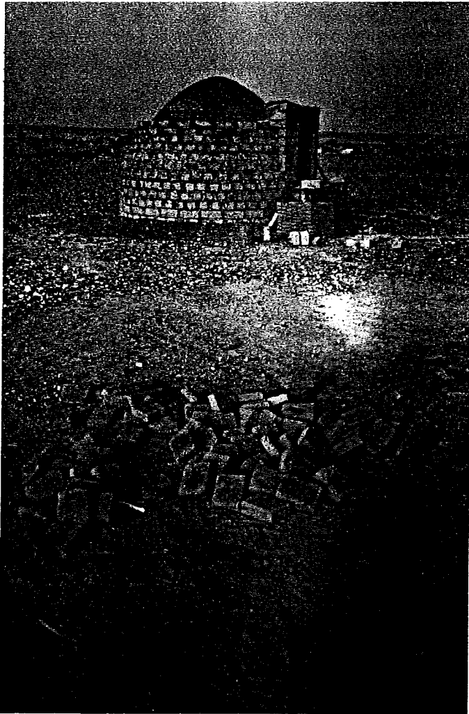
Photo 12: "Spontaneous" construction, Tchirozérine.
