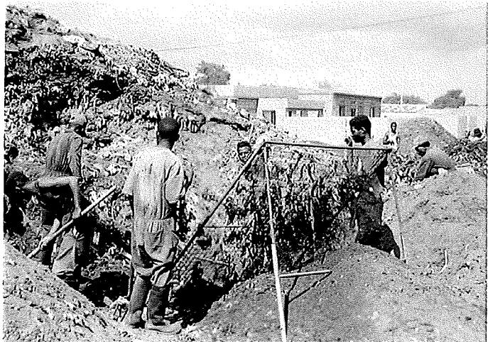
Figure 6 The results of the waste separation process: piles of sand were collected behind the wire screen while solid waste remained in front.
