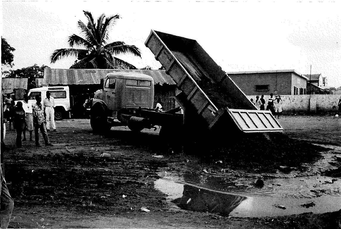
Photo of Sanitary Landfill Project
