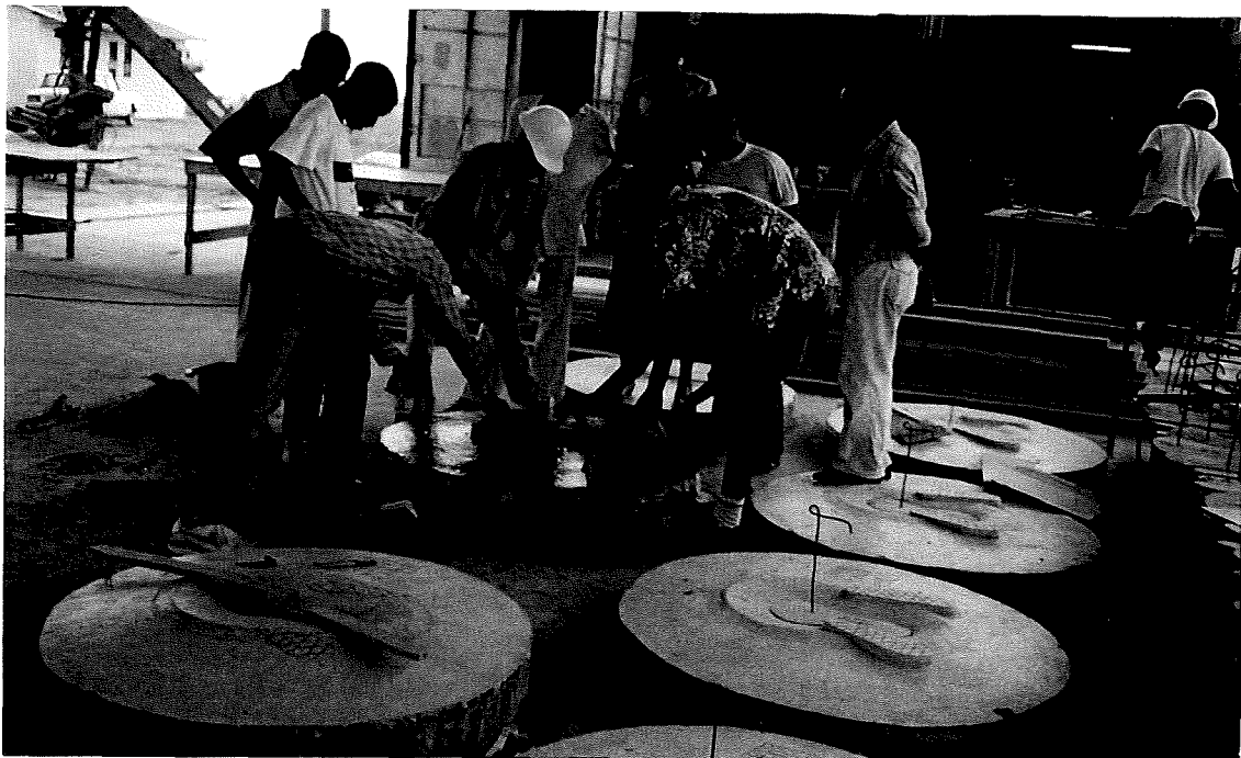
Photo of Latrine Production Workshop
